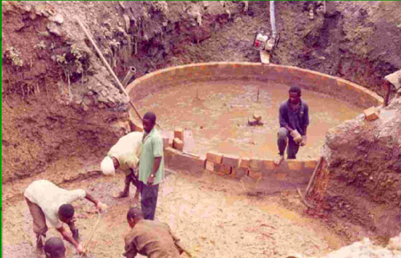
BIOGAS DIGESTERS UNDER CONSTRUCTION IN A WATER LOGGED AREA
