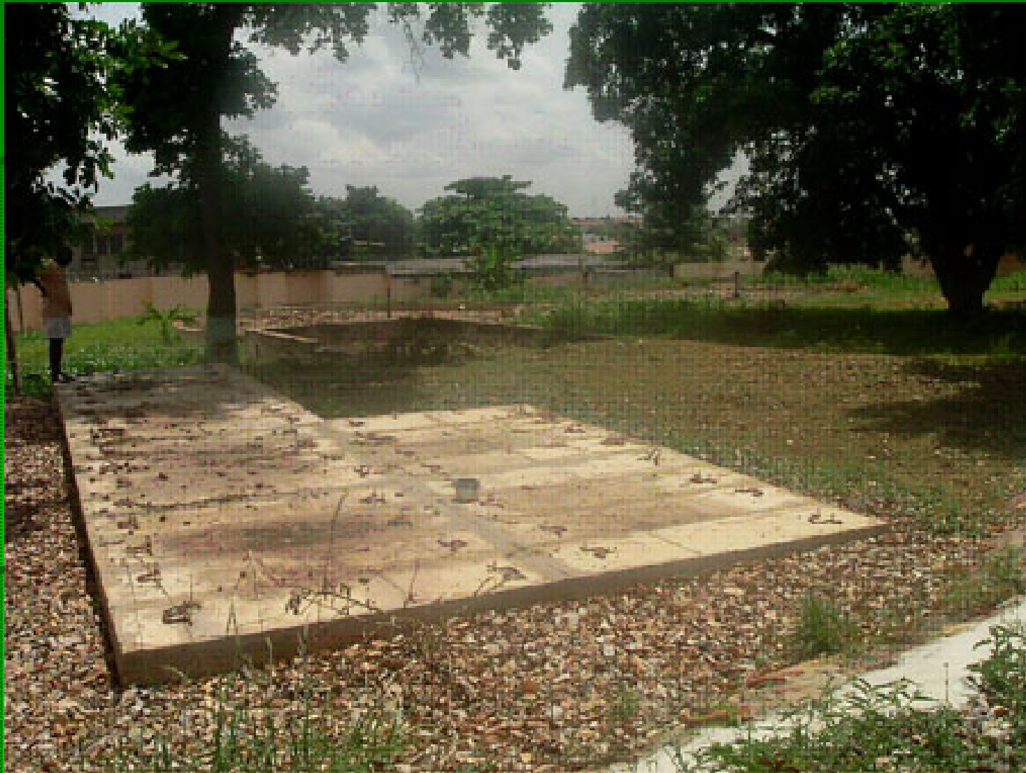
A COMPLETED FILTRATION BED
